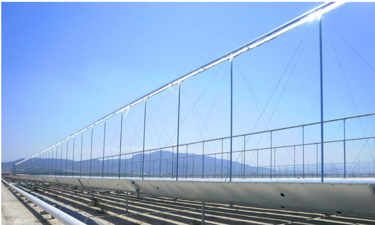
Figure 1 Supernova Collector, generating superheated steam achieving temperatures above 500°C
