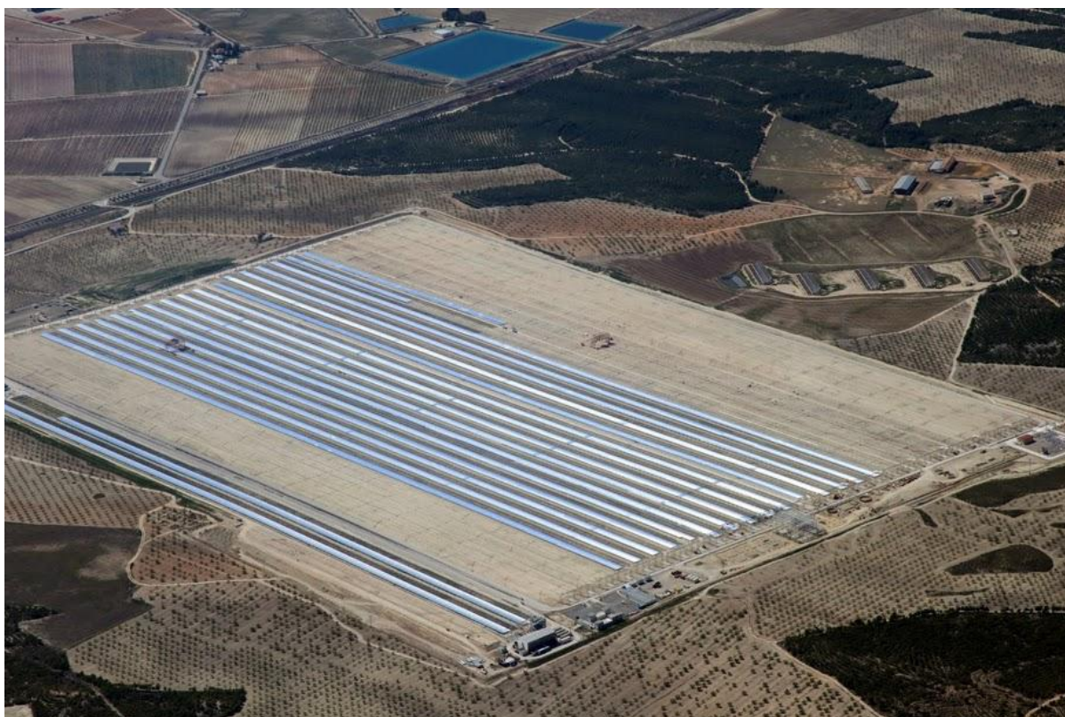
30 MW e1 solar power station PE2 under construction (Picture NOVATEC SOLAR)
